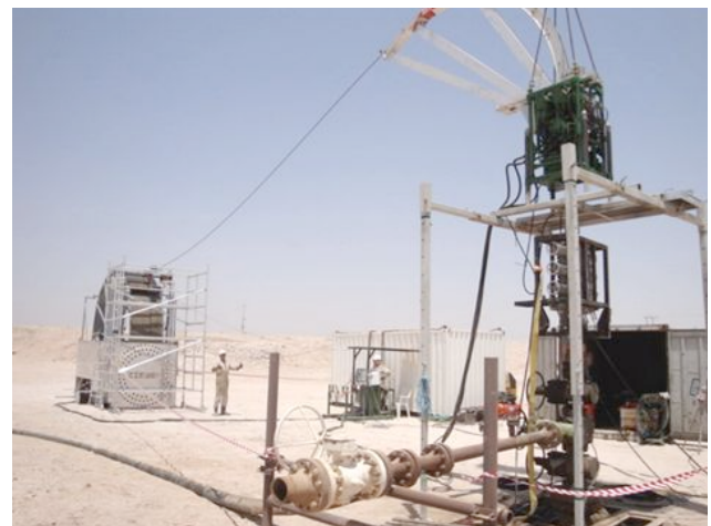
Fig. 3 – The surface system rigged up on land well in Oman
