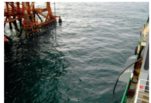
DeepFlex pipe flowing produced fluids from a production platform to the Bourbon Opale in a well test
